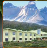
Puerto Natales Lodge Torres del Paine
